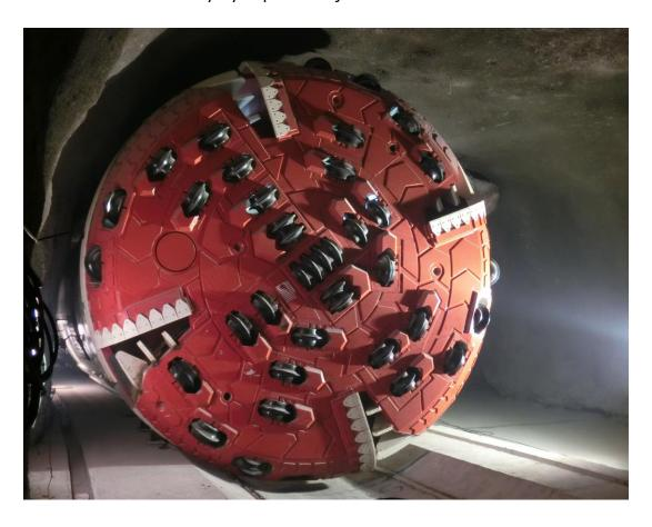
After its assembly and sliding through the launching addit, the TBM commenced its round the clock boring in July 2015. As of 31<sup>st</sup> July 2016, the TBM driven by the Tunnelling Contractor SELI Overseas S.p.A. completed 6,442m. In the last three months, the machine has registered sustained advances of 806, 824 and 1,004 meters. For this diameter of shield machine and especially when evacuating the rock by Rolling Stock, these figures are believed to be a record in South East Asia.
